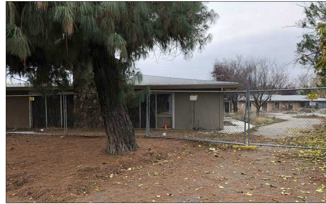
18 LOOKING WEST AT SITE FROM FRONT SETBACK
