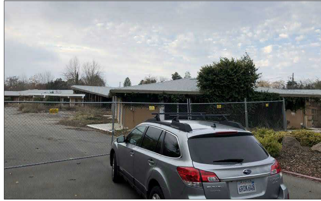
6 LOOKING WEST FROM DRIVEWAY
